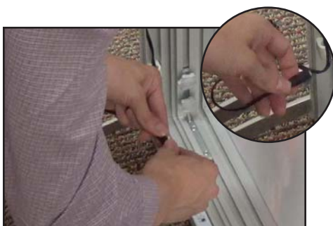
Disconnect cord extension from driver.
