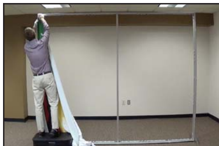
Insert Silicone Edge Graphic (SEG) into top left corner of the frame.
