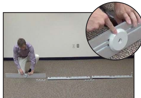
Lay out 3 extrusions with pre-installed foot at the bottom.
