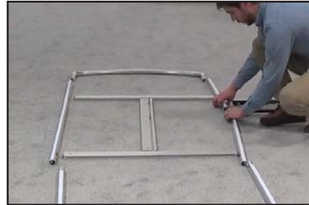
Insert tube until button lock engages on the other side.
