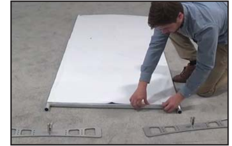
Continue attaching the liner with some tension.
