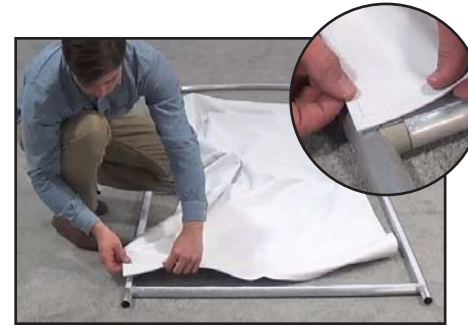
Attach liner to Velcro® at the BOTTOM corner and continue around the frame.
