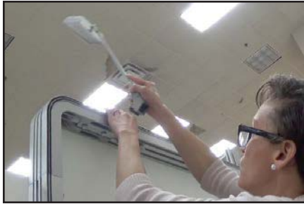
Connect lights to the top of the frame.
