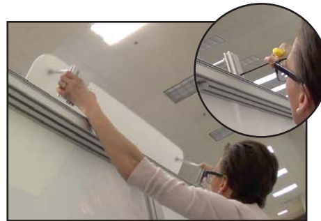
Lift header and insert mounting plates into middle channel atop the frame. Lock with hex wrench.
